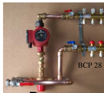
BCP28 Thermostatic Valve, variable from ambient to a maximum of 65°C as shown on the red adjustable cap.
